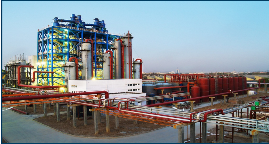
ZAO ZHUANG NEW GAS COMPANY (ZZ) – Completed December 2007
